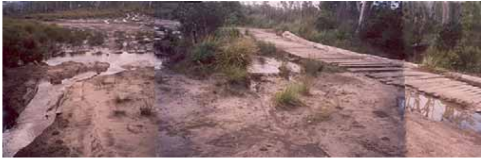
Figure 1: Formed Creek Crossing
