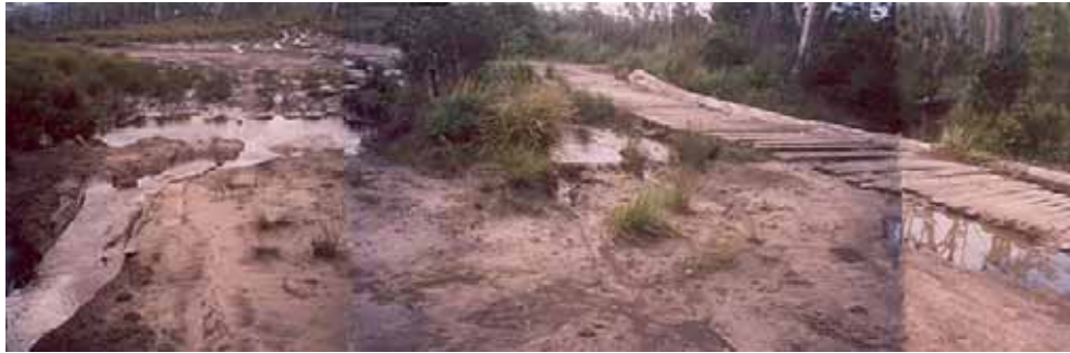
Figure 1: Formed Creek Crossing
